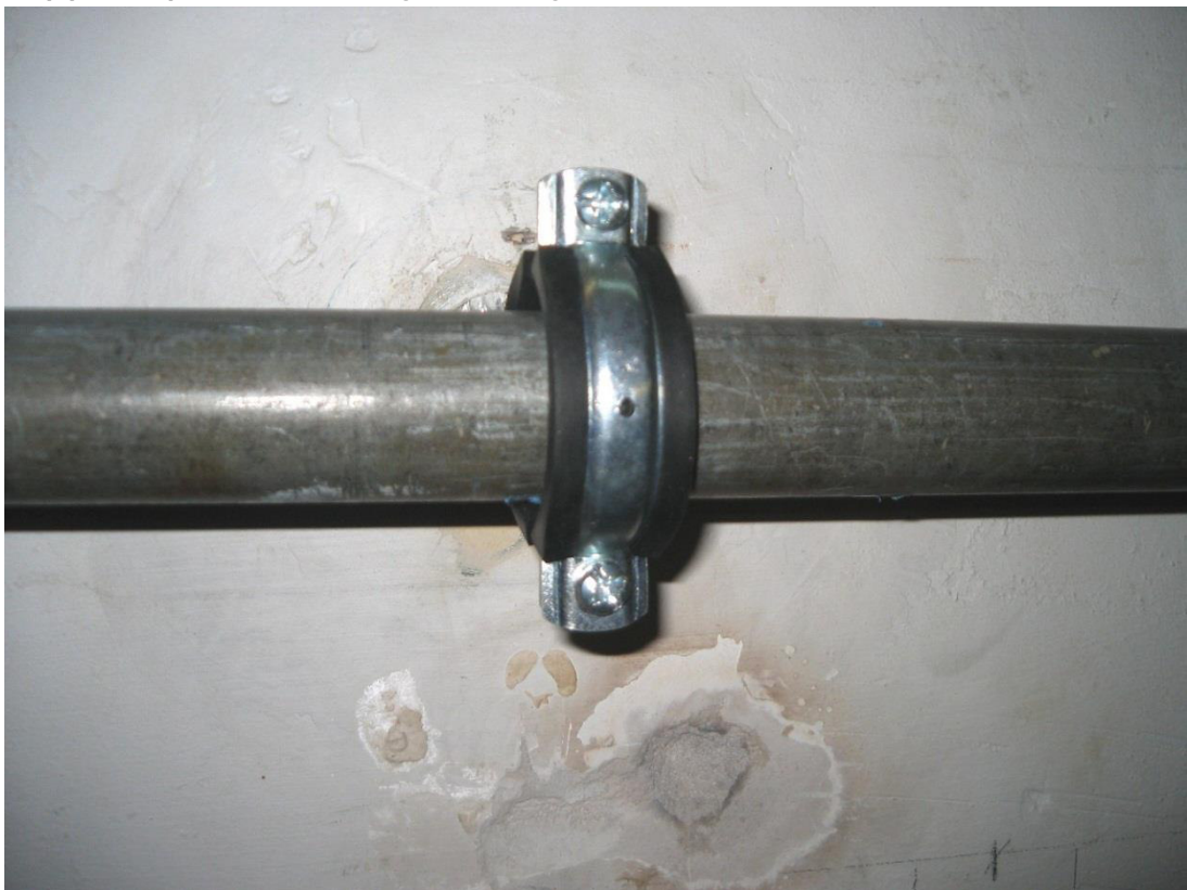
Fig. 2: Screw-pipe-clamp DÄMMGULAST® gelb, (Kreuzgeometrie), M8/M10, 1" (32-38mm)
