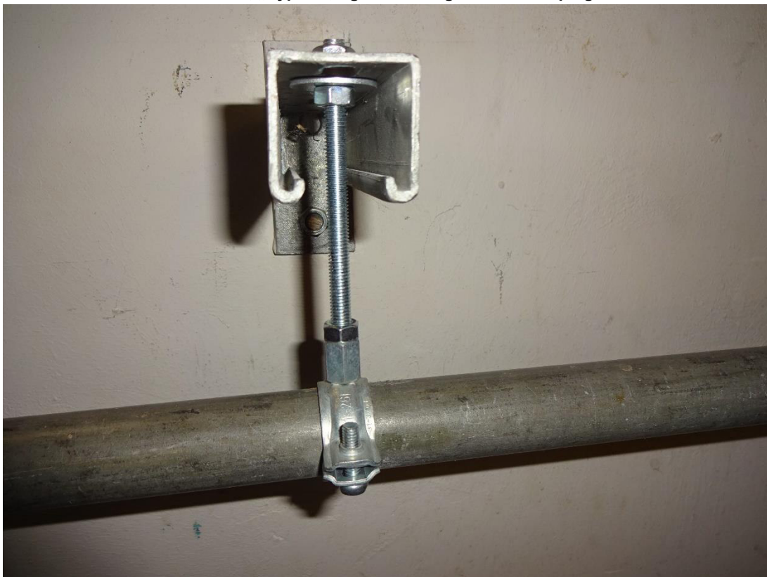
Fig. 2: Reference meas.: DÄMMGULAST®, „Type 1“, rigid fastening without damping element
