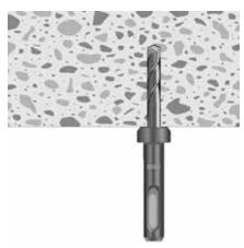
Drill with the MPC-Headed drill.
